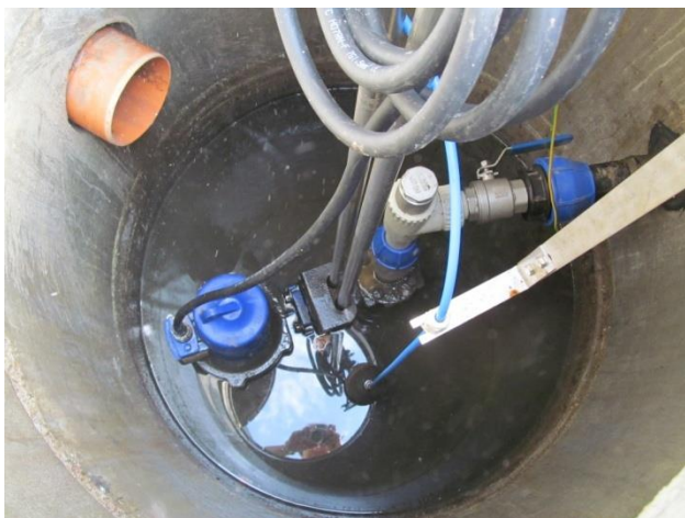
Figure 2. Domestic sump pump with centrifugal submersible pump
