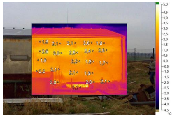
Figure 9. North façade of poultry house 2 - part 2
