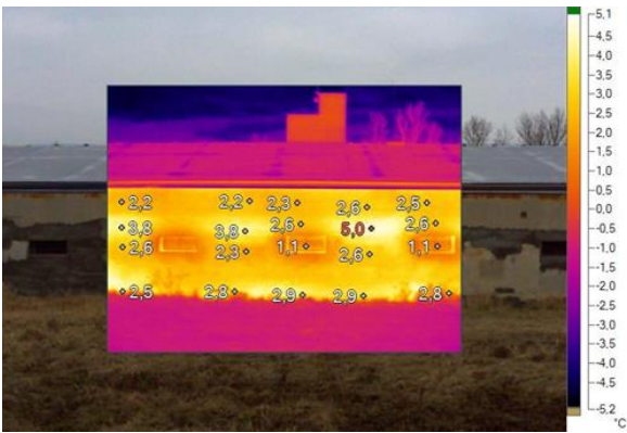
Figure 12. South façade of poultry house 2 - part 2
