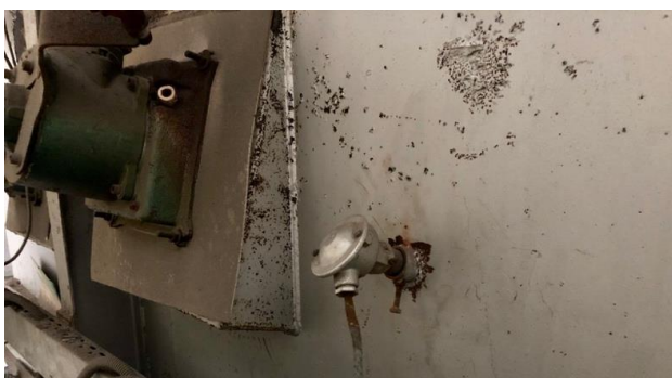
Figure 2. Installation of the resistance temperature sensor Limatherm Sensors TTSC-22 in the gas melting furnace KOV 010/1998
