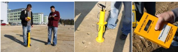
Figure 7. Testing the degree of compaction of earth plane by Clegg Impact Soil Tester with indicating the CIV reading
