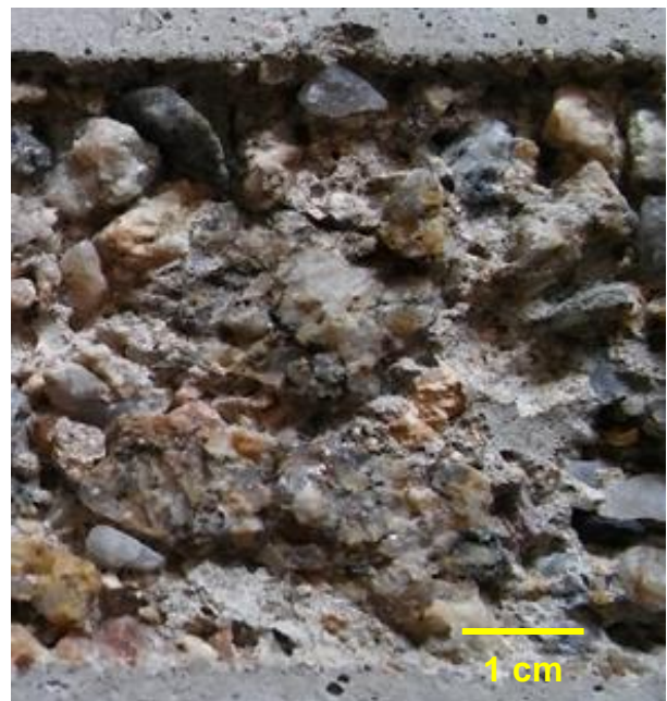
Figure 4. Detail of cut in concrete made by rotating water jet, pressure 210 MPa. Concrete C50/60, CEM 42.5 R, siliceous sand (0-4 mm) and
