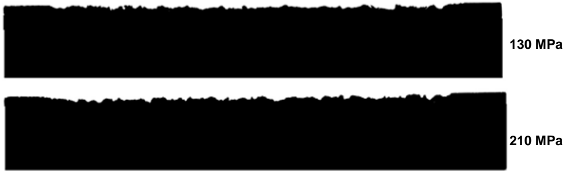
Figure 2. Reliefs of the concrete surface created by rotating WJ, 2 nozzles in rotary head, water pressure 130 and 210 MPa. Concrete C40/50
