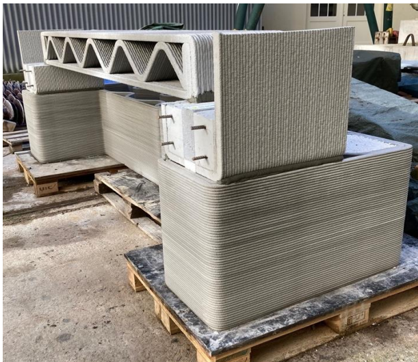
Figure 8. Printed wall and truss beam
