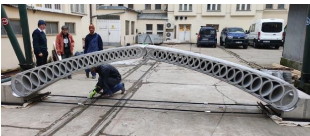
Figure 21. Setting the footbridge into final position
