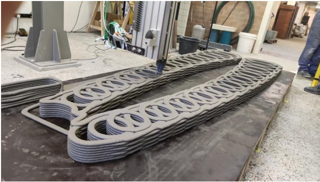
Figure 19. Printing the footbridge.
