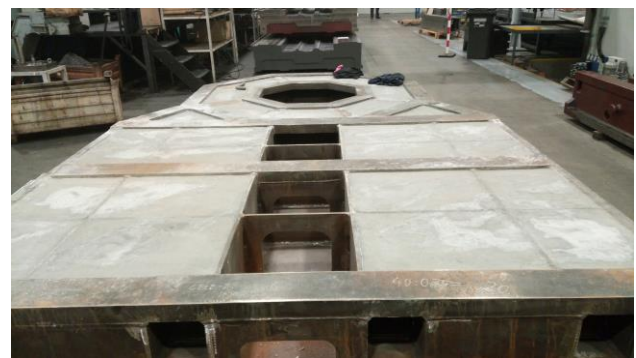
Figure 1. Steel-concrete bed being filled with high-strength concrete
