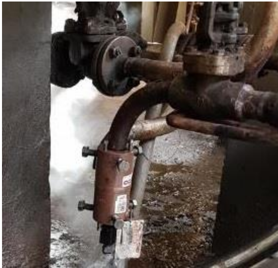
Figure 22. Stopping leakage using PLIDCO Weld+End blanking sleeve [SEPS 2022]
