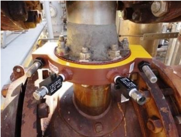
Figure 8. PLIDCO Flange Repair+Ring flange sealing ring [SEPS 2022]
