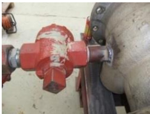
Figure 24. Welding the throat on and drilling through it during operation [SEPS 2022]
