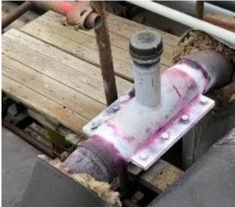
Figure 28. Sleeve with a throat after the works finish during operation [SEPS 2022]
