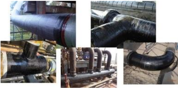
Figure 6. Composite bandage installation [SEPS 2022]
