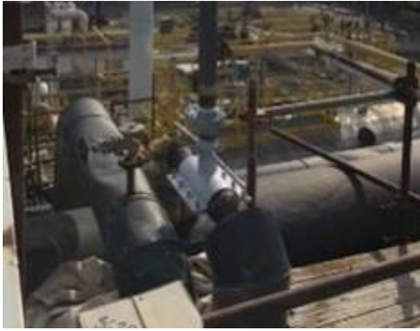
Figure 27. Installation of the sleeve with throat and exhaust [SEPS 2022]
