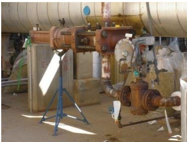
Figure 19. Boiler water pipe closure (Boiled Feed Water) DN80 [SEPS 2022]
