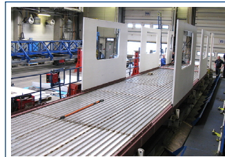
Figure 12: Test-fitting of side walls onto the main frame
