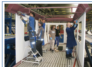
Figure 14: Application of adhesive to the purlin joints on side walls
